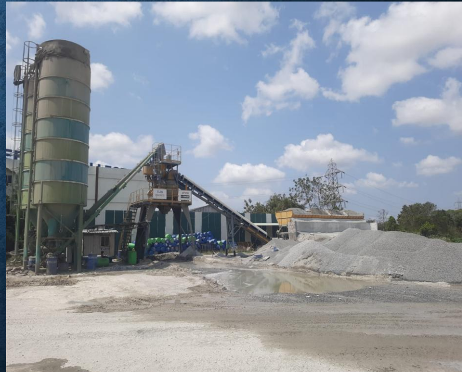
Ready Mix Concrete Plant
